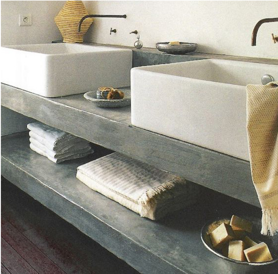
mobile lavabo in muratura
